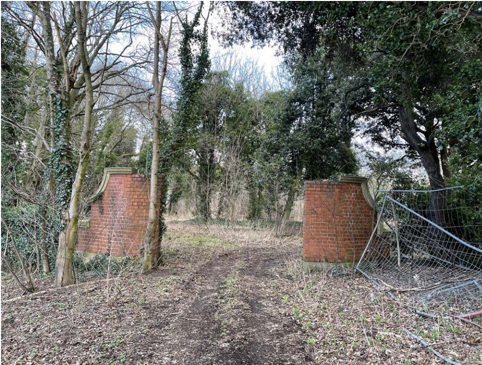
Fig 30: Sudbrooke Holme Forcecourt gateway - piers and boundary walling.
