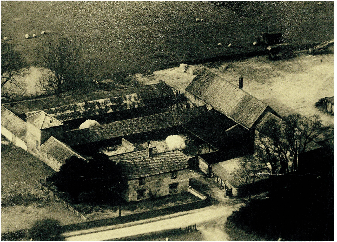
CHURCH LANE MANOR FARM
