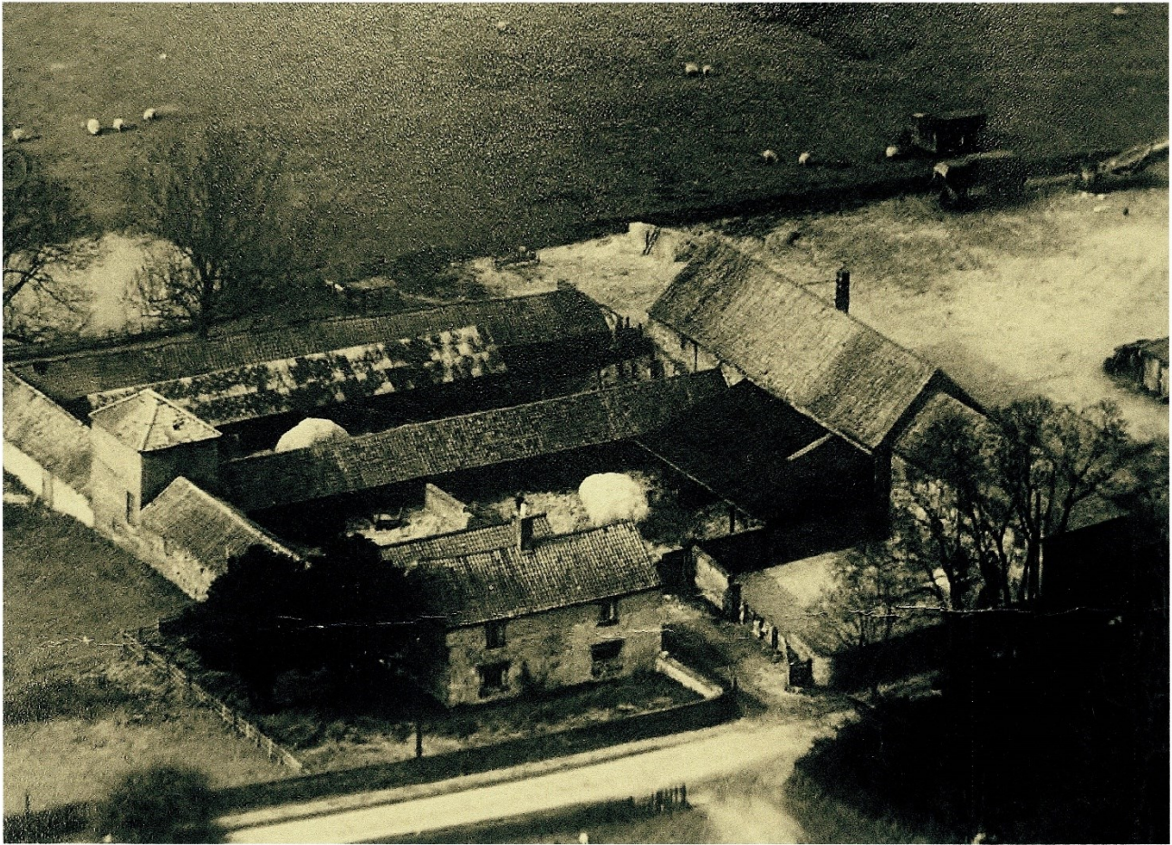
CHURCH LANE MANOR FARM
